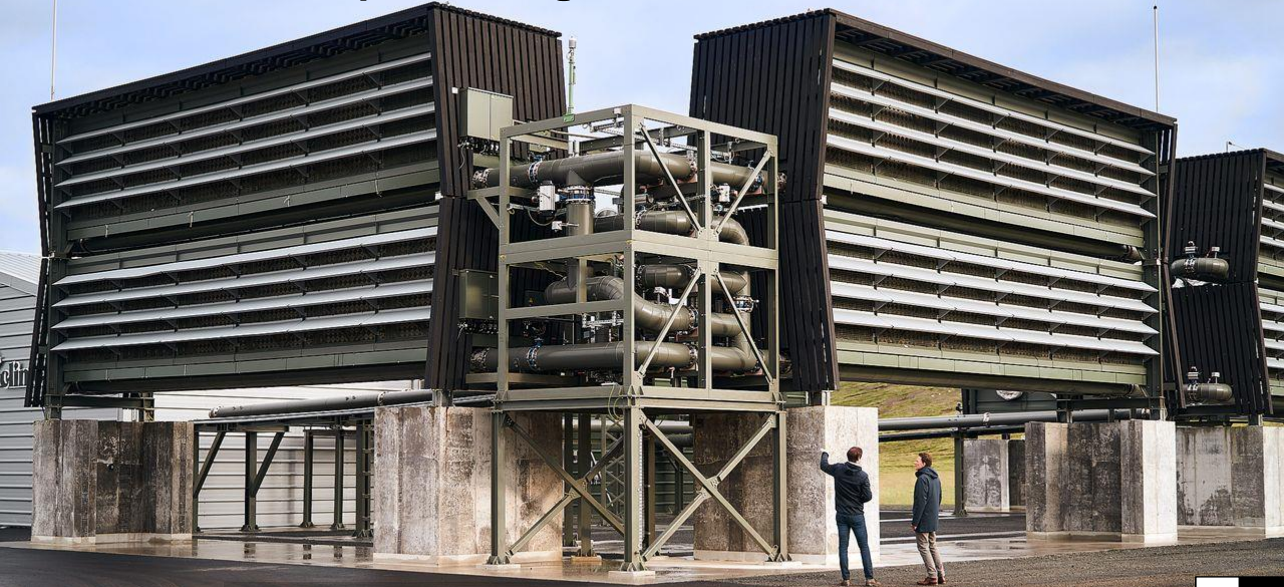
ORCA Carbon Capture Plant, Hellisheiði, Island 4 kt CO 2 /a
